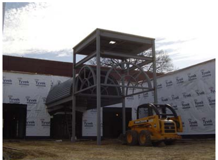
The West entrance tower under construction.
