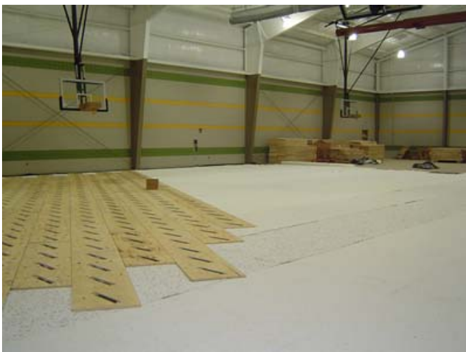
Gym floor installation is currently underway.
